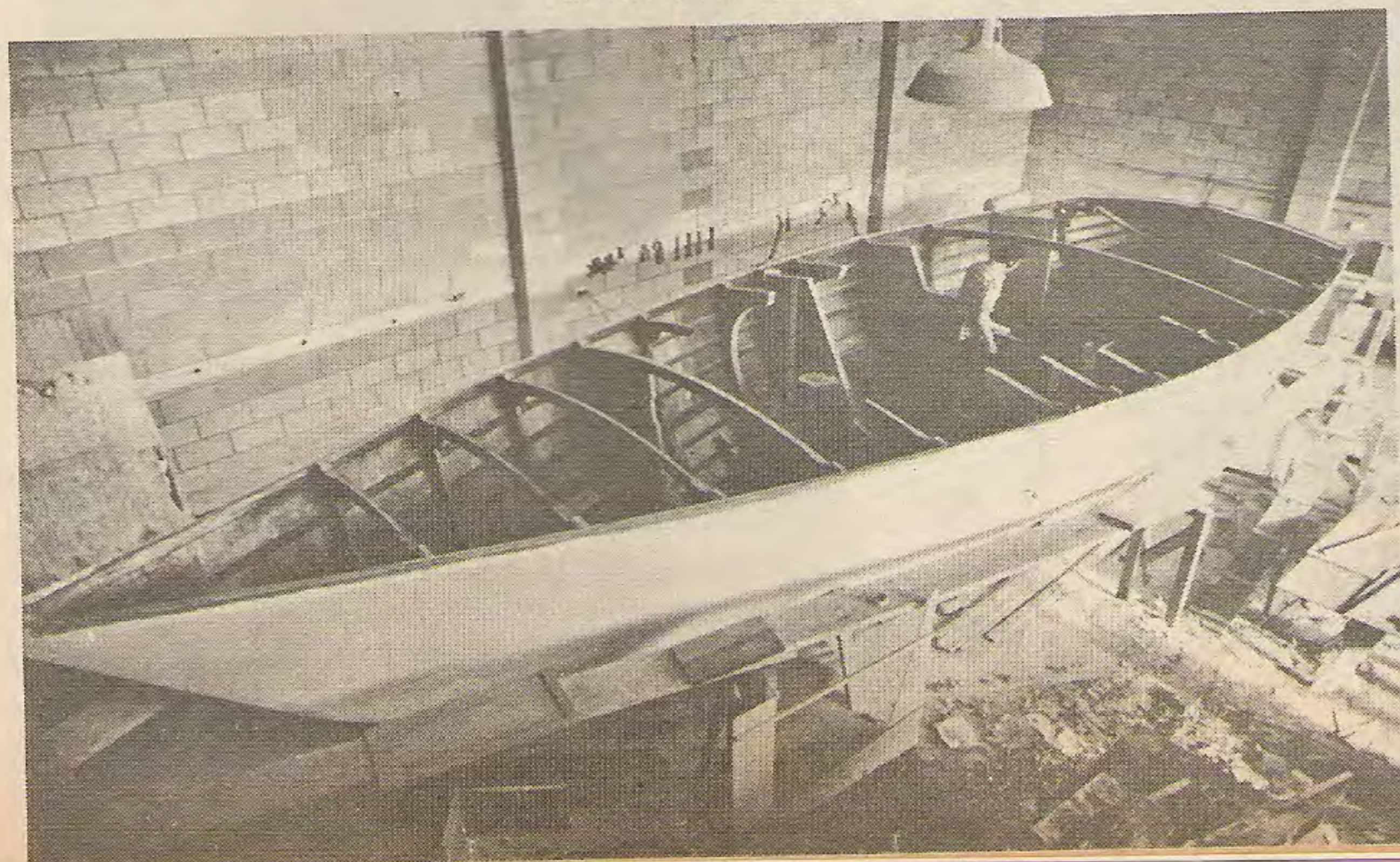
The hull after turning
